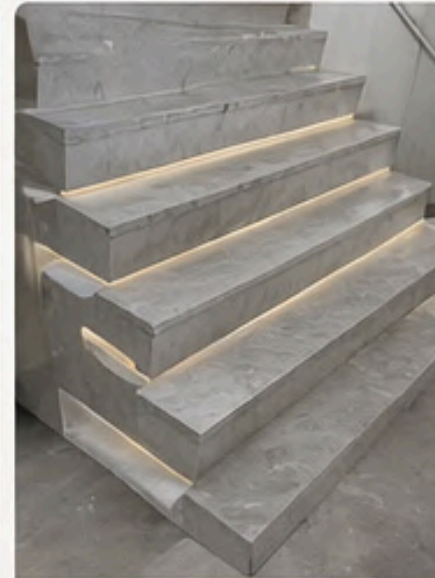
STAIR & FLOORING ELEMENTS
